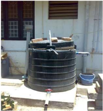
Kitchen waste Biogas Plant
