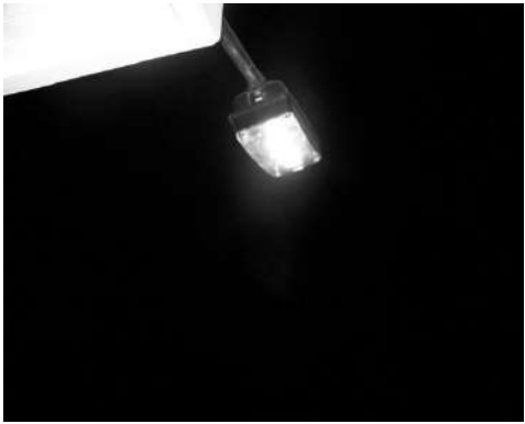
LED solar lightings
