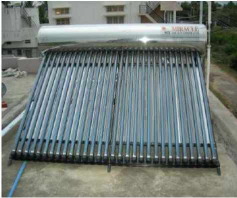
Evacuated Solar Water heater
