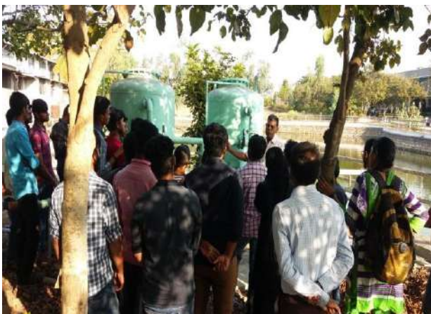
Dr. Sreepathi showing water treatment process installed at college campus.
